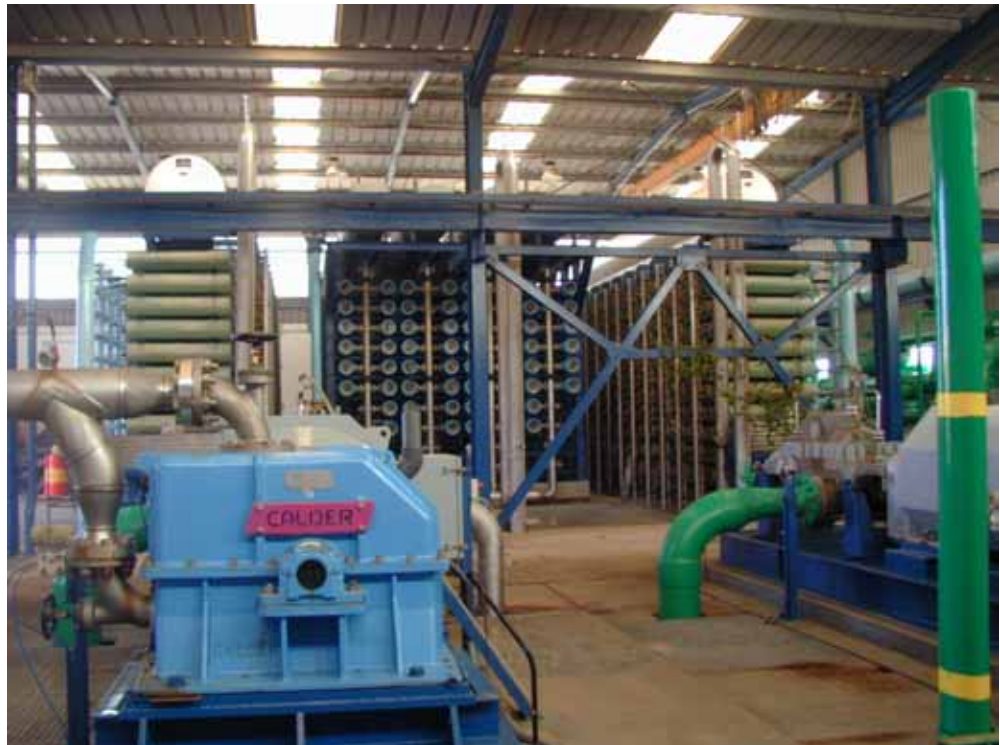
Train 2 at the Agragua, Spain, seawater reverse osmosis facility (shown as the middle train in the background of this photo) was retrofitted with FILMTEC™ spiral wound elements. The high pressure pump is shown in the foreground. (Photo courtesy of Agragua Desalination Plant)
